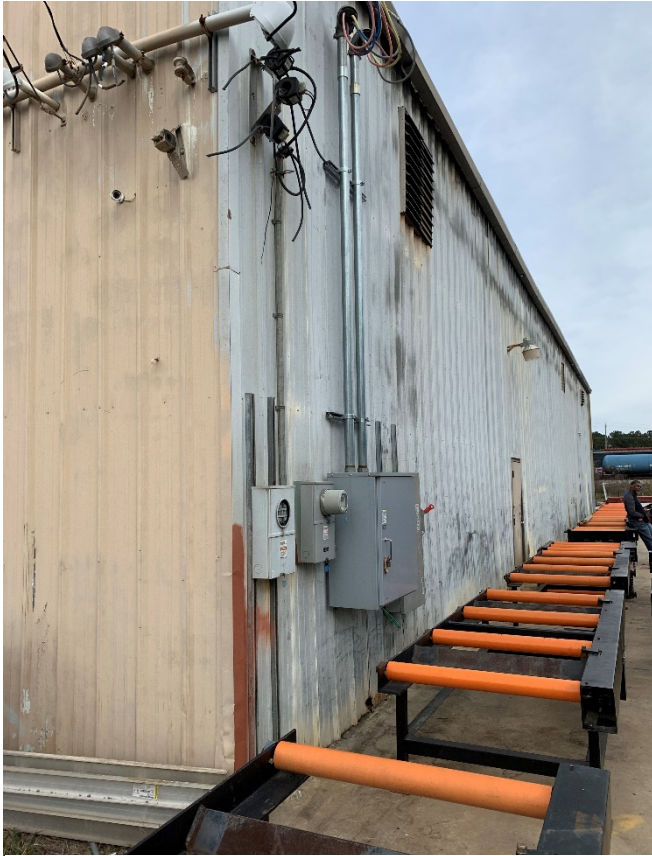
Figure 3: Future site of the building addition and conveyors
