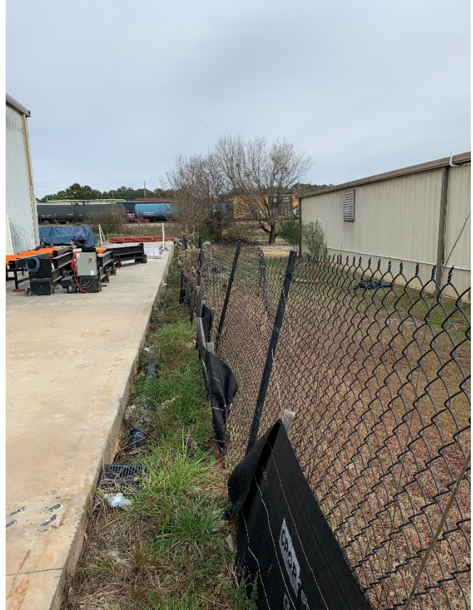
Figure 4: Existing fence on southside of building
